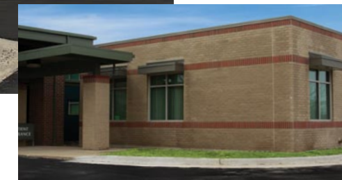
The building project added space for the Business Department.
